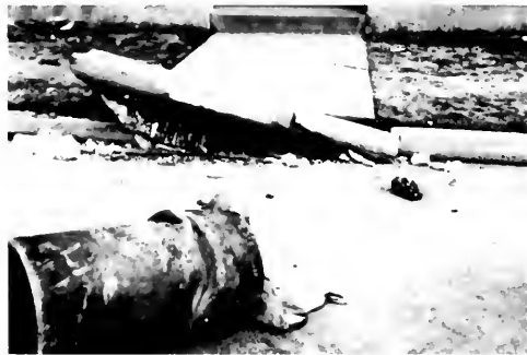
Photo 14. Compressed section of gas pipe removed from the main line across the thrust faulting near Glenoaks Boulevard, San Fernando. Note ejected concrete curb.
